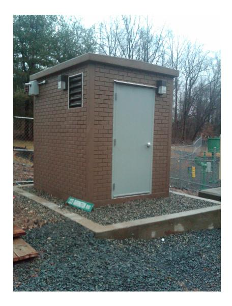
Here is a small precast building with a brick finish that was used for electrical panels at a pump station. The building was specially designed for high winds and bullet protection. The contractor added the color staining and fixtures on site.
